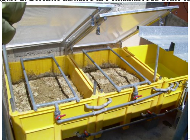
Figure 2: Biofilter installed in Fontanafredda demo farm
