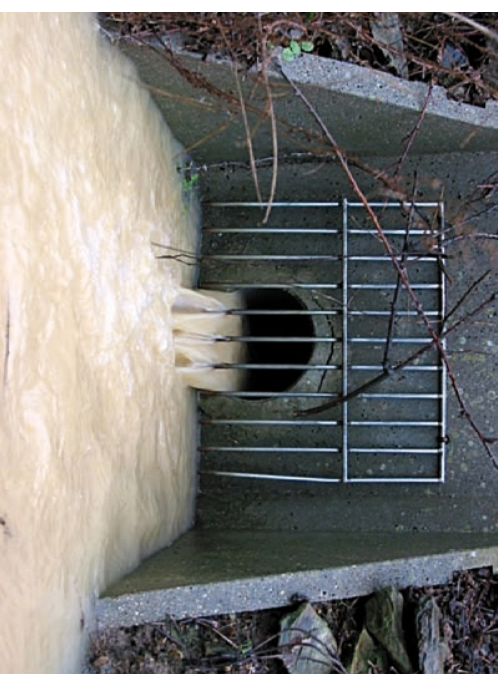
Figure 9: Subsurface drainage outlets
