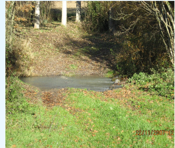
Road crossing a stream
