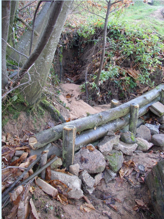
Gully control and dispersion fascines (Beaujolais vineyard)
