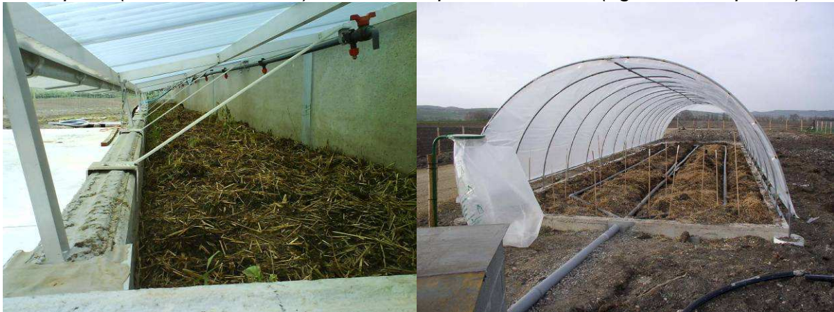
Fig. 23 & 24: Distributing the contaminated liquid over the surface by means of spraying nozzles (left, source POVLT) or a circular perforated pipes (right, source Bayer CropScience).
