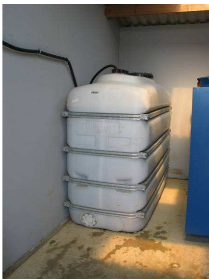
Fig. 18 & 19: example of a 4000 l. PE buffer tank above ground and a 5000 l. concrete buffer tank beneath the filling and cleaning place with separation valve for rain water (source: pcfruit).
