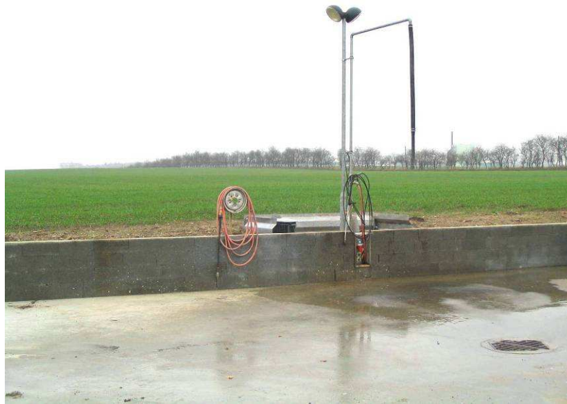
Fig. 15: Separate concrete filling and cleaning area with filling and cleaning equipment, which drains contaminated liquids to the bio purification system (source: DAAS).
