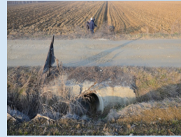
Shortcut to river by pipe
